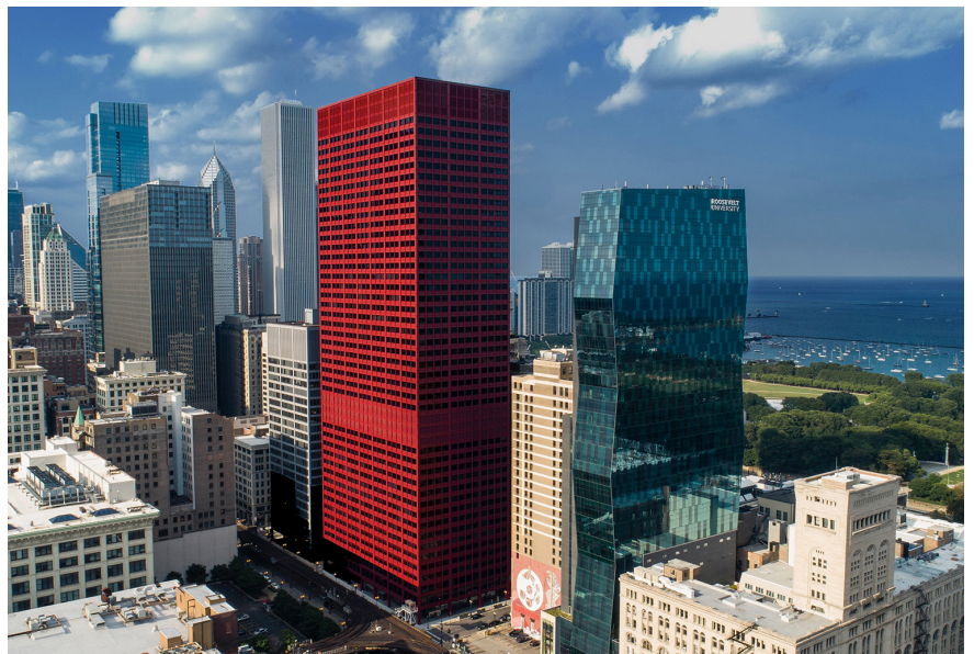
„BIG RED“ PRIME OFFICE TOWER – CHICAGO
